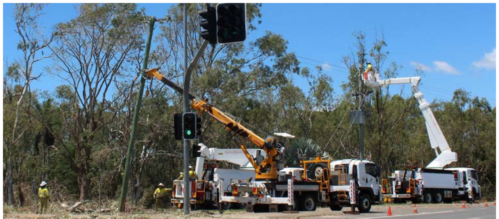
Ergon Energy staff did a fantastic repair job.
