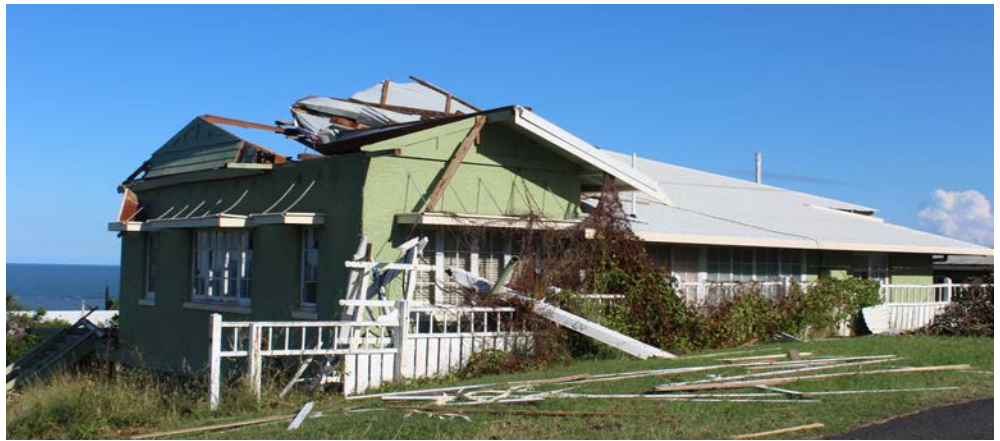
More than 1,500 homes were damaged in the region.
